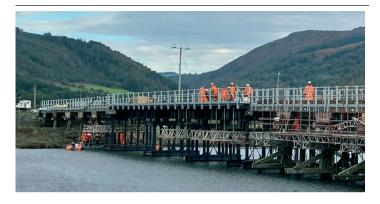
Refurbishment of the Dyfi Bridge was completed last November. Parts of the wooden structure were replaced with Glass Reinforced Plastic (GRP) resin. About 77 tonnes of timber removed from the structure have been recycled, and around 90 metres of track panels donated to the Gwili Railway. Photograph: Network Rail.
